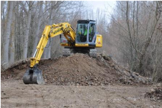
Figure 8 . Example of a measure included in the Órbigo River Restoration Project (Douro River Basin): removal of a useless levee.
