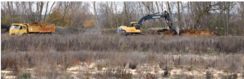
Figure 9 . Example of a civil work developed in the Esla River (Douro River Basin). The owner of the field located in the flood prone area had to undertake the removal of an old levee as a precondition for planting poplar trees.
