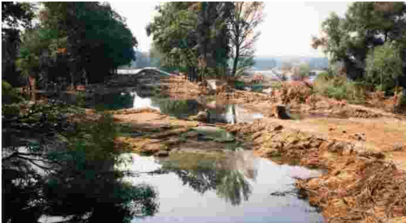
Figure 6.4 Levee Failure at the Oder 1997 near the village Wiesenau. Foreground: large scourholes in the levee axis. Background: remaining levee cross section. Trees at the landside toe hindered the levee slope inspection. On the right side: the Oder river. (photograph: R. Pohl)
