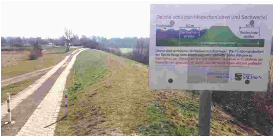
Figure 6.5 Levee at the Elbe in Dresden. View upstream from Washington st. bridge (photograph: R. Pohl)
