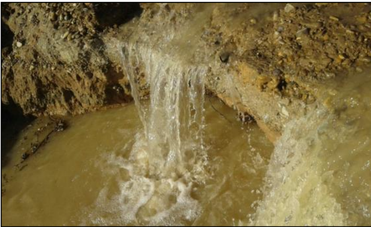
Figure 7. Seepage through a levee that may cause its collapse.
