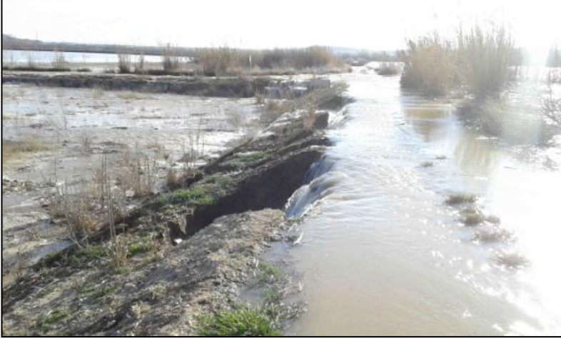
Figure 4. View of a levee during an overflow.
